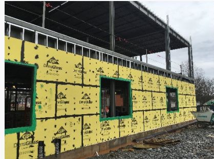
Exterior Sheathing & Air Barrier Prep Work
